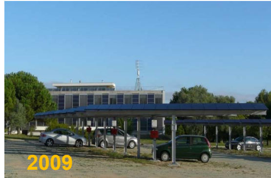
Solar XXI BIPV from LNEG
