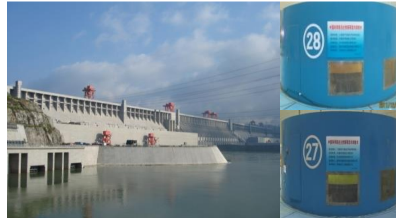
Two 700MW water turbine generator
